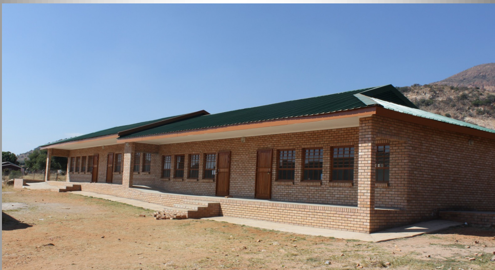
Mmanyama Primary School: Capricorn District, Construction of 1x 4 Classroom
