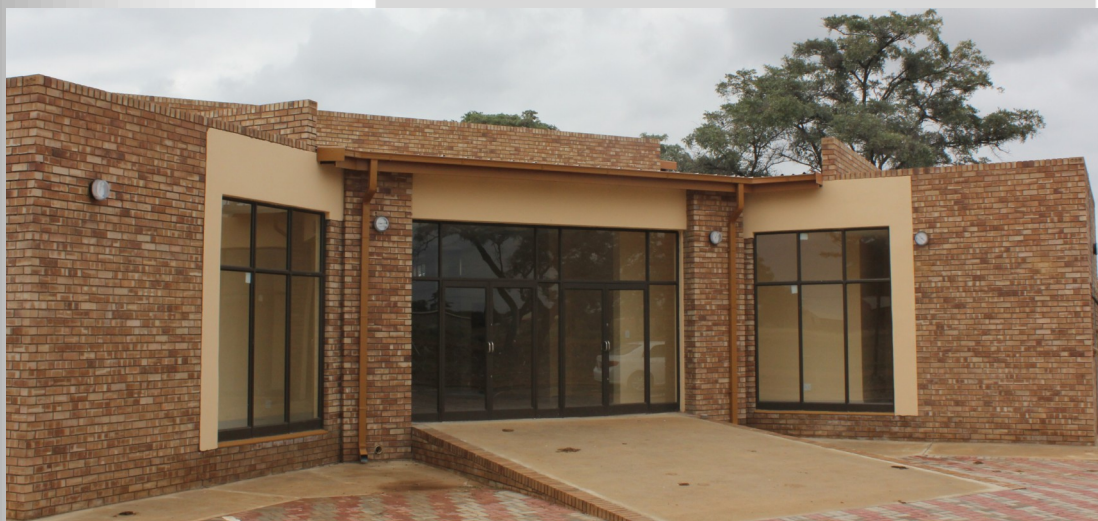
Rapotokwane : Waterberg District, Construction of Library
