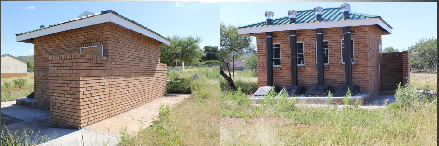
Makopi Secondary School: Sekhukhune District, Construction of 1x 4 seater envoroloo toilets block
