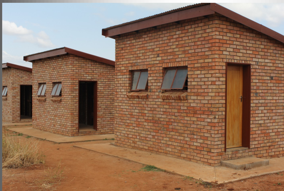
Kgati ya Moshate High School: Waterberg District, Construction of 3 x 4 seater enviroloo toilets
